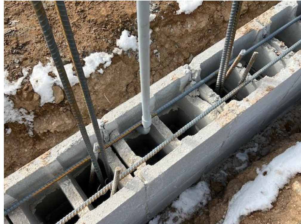
Masonry Stem Wall / Vertical and Horizontal Rebar / Electrical Conduit
