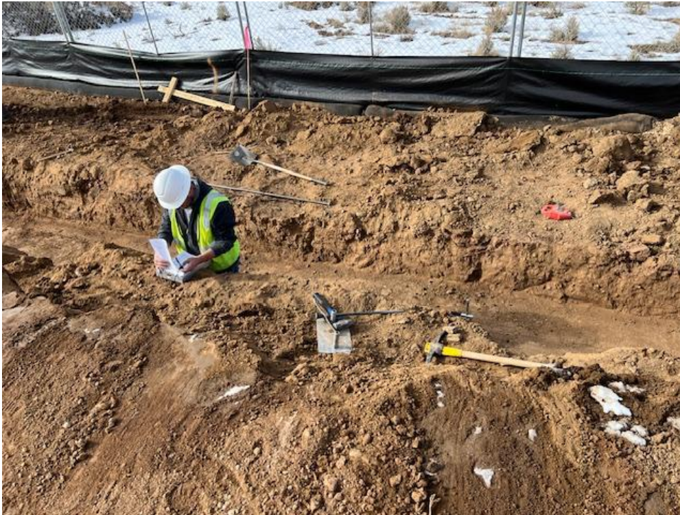
Taking Soil Density Tests at Masonry Retaining Wall Trench
