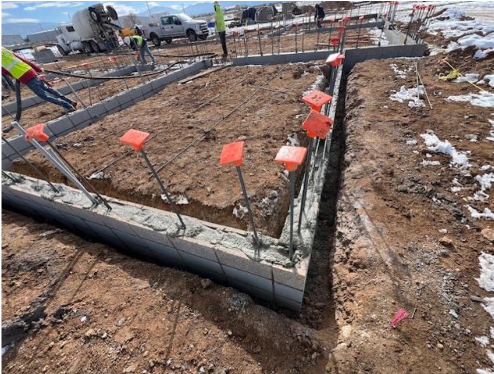
Masonry Stem Wall and Burnished Block / Rebar / Electrical Conduit
