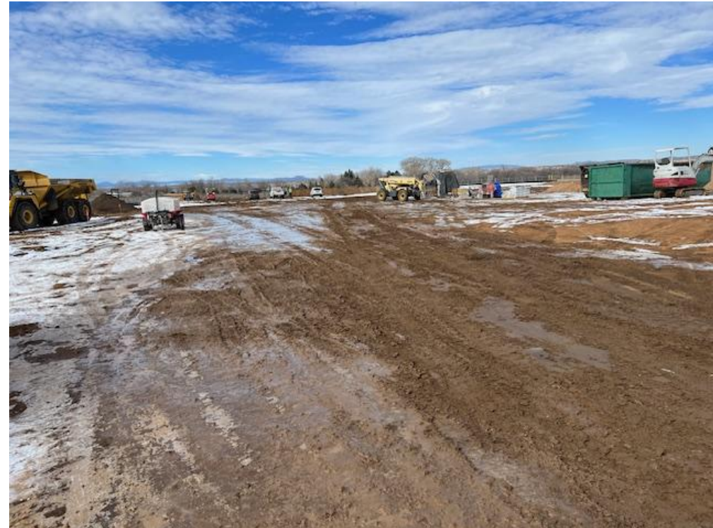
View of Site Looking North From Entrance off of Salazar
