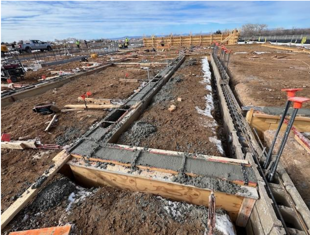
Concrete Stem Walls with Fresh Concrete Placement / Rebar
