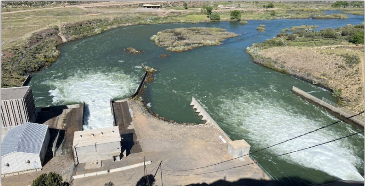
Navajo Dam showing the release of 4,000 cfs under the Jicarilla Apache Nation lease in 2023. Photo: U.S. Bureau of Reclamation.
