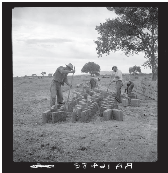
Making adobe bricks. Bosque Farms project, NM. These bricks are to be used in construction of the new school building.
