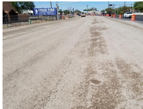
(b) Compacted base
