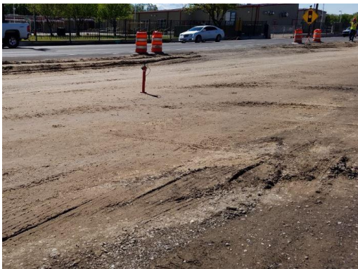
(a) Compacted subgrade
