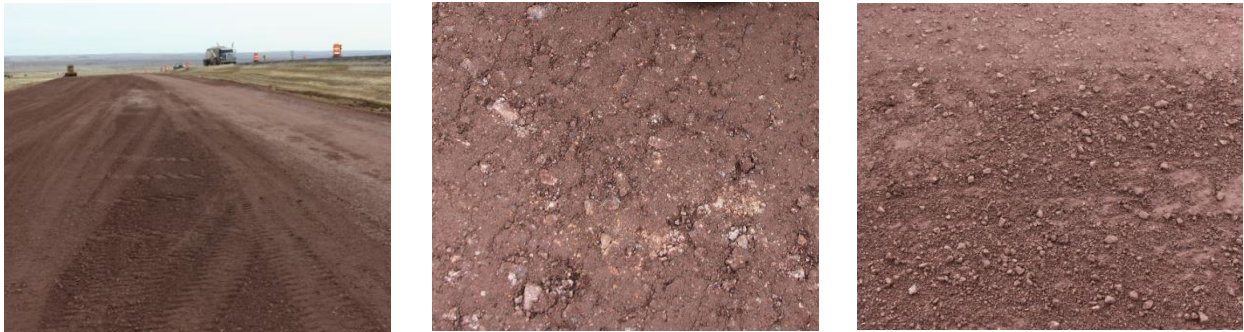
FIGURE E-1 Compacted base course of US491
