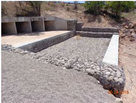
Combination wire-enclosed riprap and gabions below CBC apron. Location unknown.
