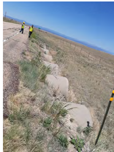
No channel evident– There is no visible characteristics associated with a dry arroyo. Vegetation is uniform throughout. Flow comes only during heavy or long duration rains as sheet flow. Location on left is unknown. Location on right is on NM 104, between Las Vegas and Trujillo, San Miguel County.
