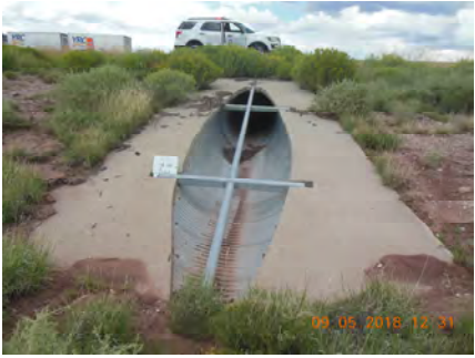
Metal culvert, with safety grate. Location is unknown.
