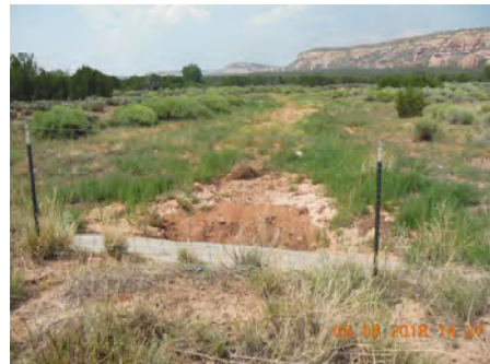
Channel above could be described as 'weeds/ debris'. Heavy weed growth on channel is due to a wet summer monsoon season. The same culvert is shown below looking at inlet. Location is on NM 53, east of Zuni, McKinley County.
