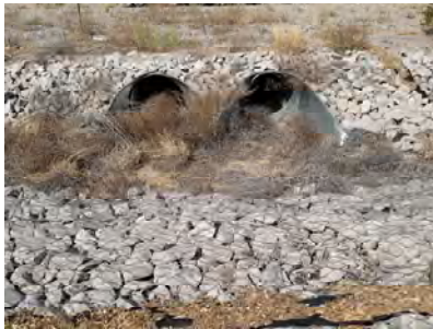
Wire-enclosed riprap
