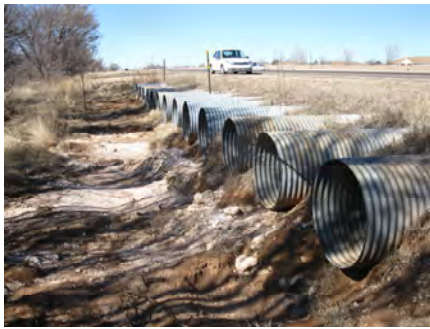
Culvert outlets above show minor scour (1 to 3 ft. depth). Location on left is on US 60 near Cannon AFB, Curry County. Location on right is on US 82, MP 136.0, Eddy County.
