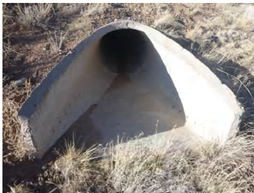
Concrete culvert pipe below
