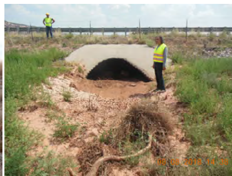
Channel above could be described as 'weeds/ debris'. Heavy weed growth on channel is due to a wet summer monsoon season. The same culvert is shown below looking at inlet. Location is on NM 53, east of Zuni, McKinley County.
