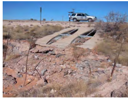
Culvert outlets above show minor scour (1 to 3 ft. depth). Location on left is on US 60 near Cannon AFB, Curry County. Location on right is on US 82, MP 136.0, Eddy County.
