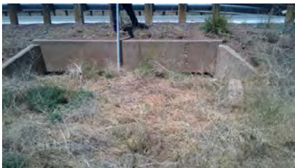
Greater than 90% silting
