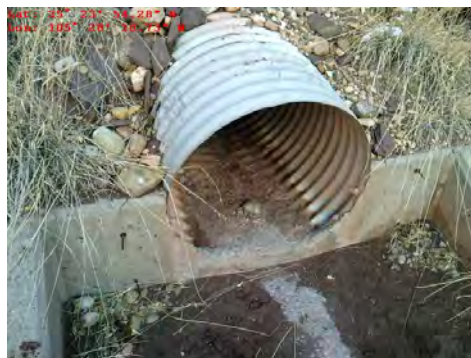
Minor corrosion on outside
