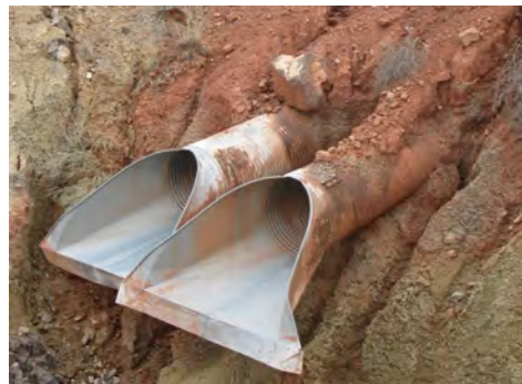
Minor corrosion on outside
