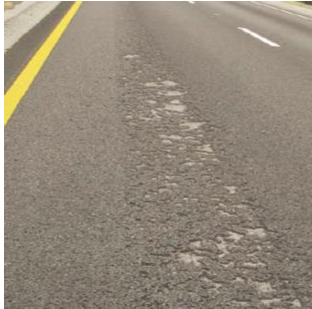
FIGURE 6 Raveling problem associated with OGFC (7)
