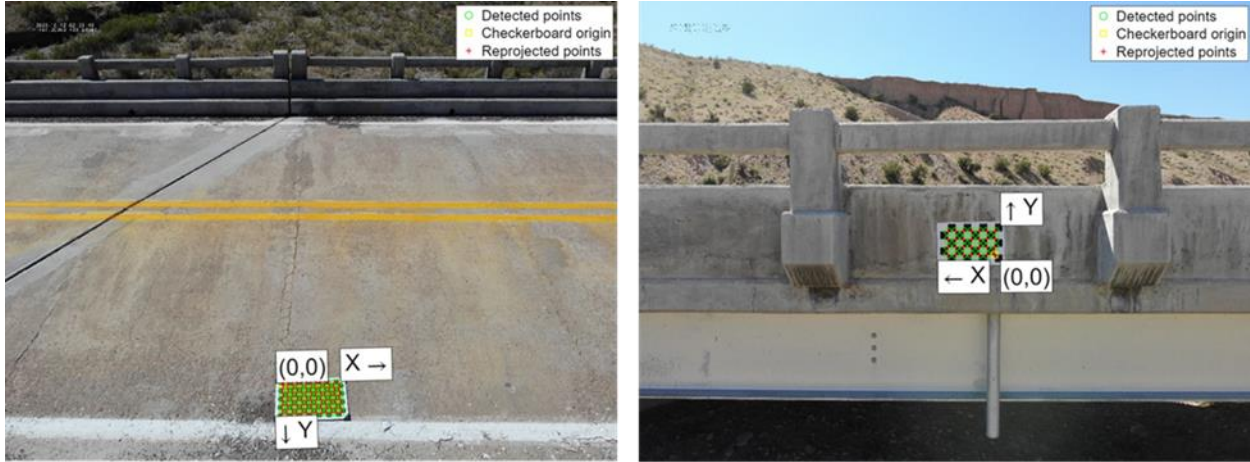
Figure 17. On-site camera calibration examples for the first bridge (NBI bridge number: 01791)
