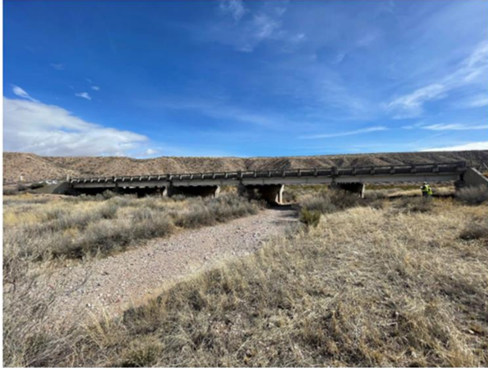
Figure 10. Profile view of the first bridge facing north (NBI number: 01791)
