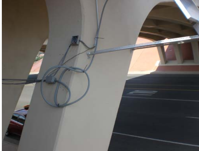
FIGURE 11 Electrical Boxes and Conduits to Pass Power to the SDAQ Using the Solar Panels.
