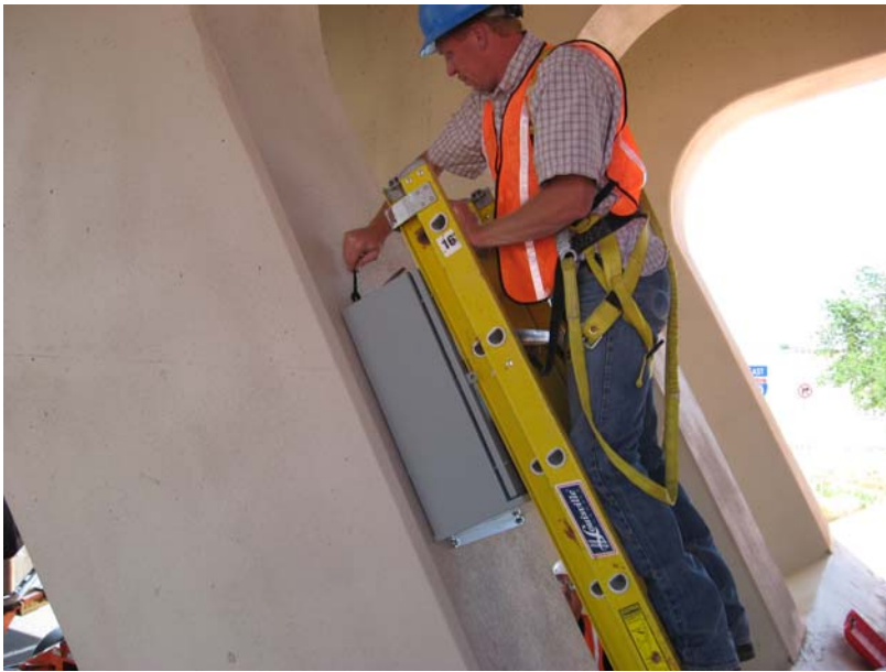
FIGURE 6 Installing of the Steel Box to House All Electrical Components at the Bottom of Bridge 7937.
