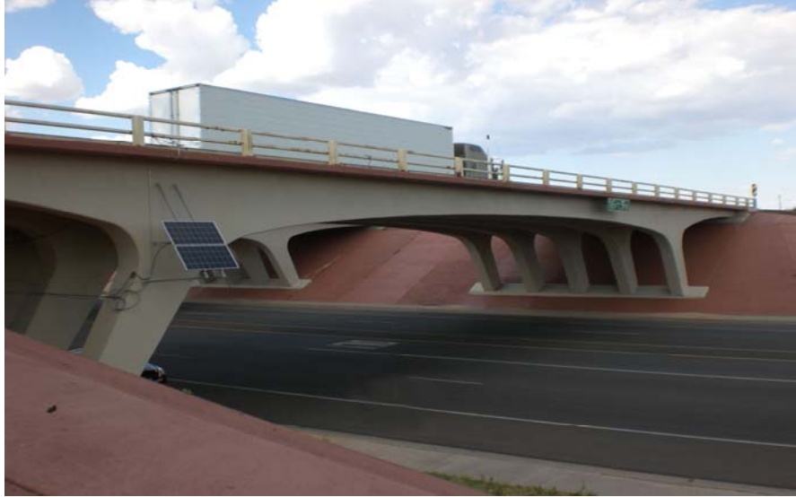
FIGURE 19 Solar Power System Installed on Bridge 7937 to Provide Clean Renewable Energy for The SHM System.
