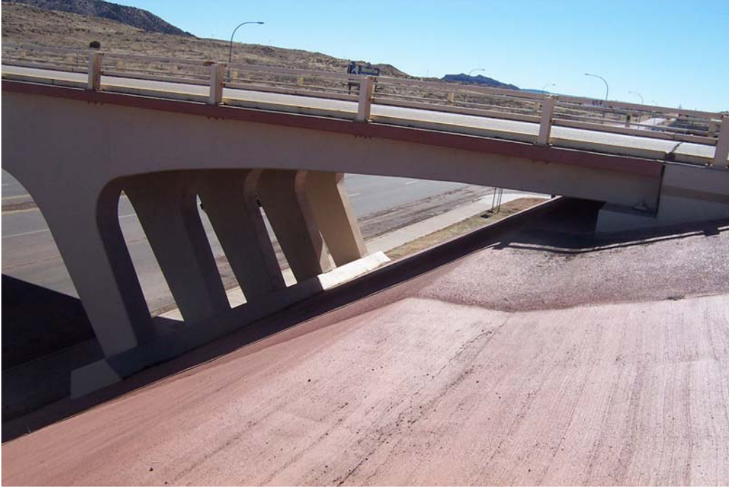
FIGURE 2 K-Frames of Bridge 7937.
