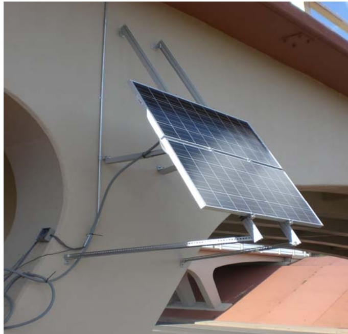
FIGURE 20 Solar Power System Installed on Bridge 7937 to Provide Clean Renewable Energy for The SHM System.
