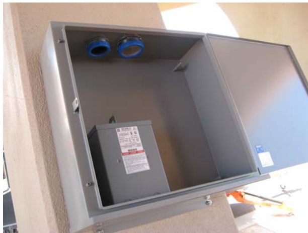
FIGURE 7 Steel Box Used for Housing the Data Acquisition System and All SHM Components.
