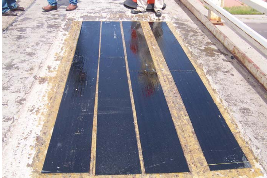
FIGURE 4 FRP Strips Installed on Bridge 7937.
