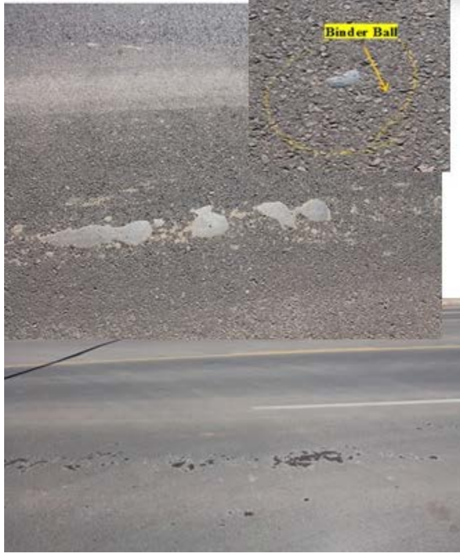
FIGURE 21 Binder Balls.
