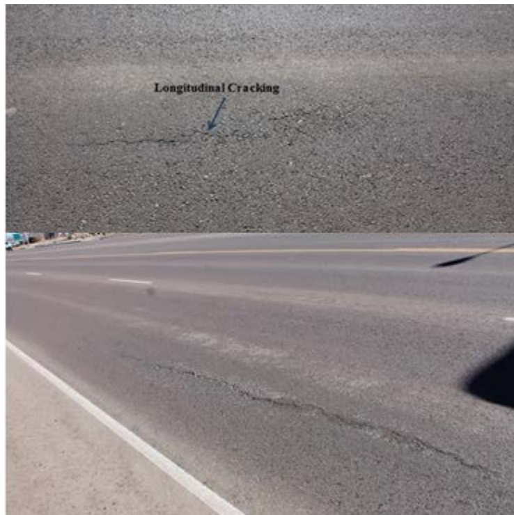
FIGURE 24 Longitudinal Cracking.
