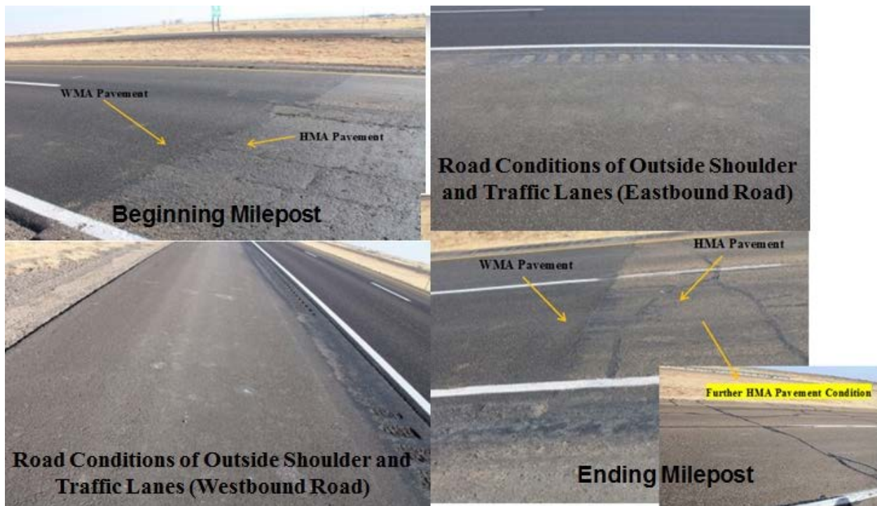
FIGURE 38 Pavement in very Good Condition from the Beginning to the Ending Mileposts.
