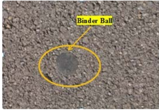
FIGURE 40 One Binder Ball Found on the WMA Shoulder.
