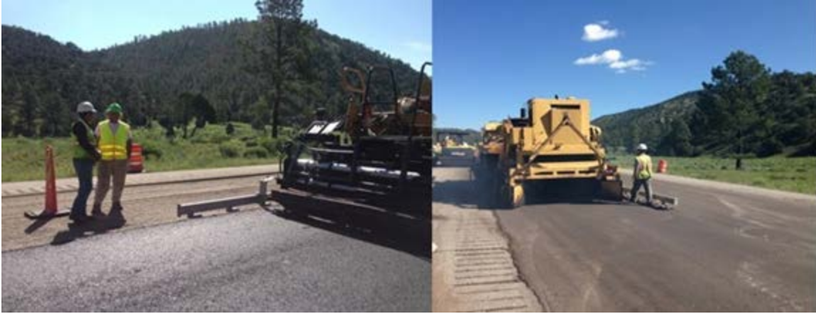
FIGURE 28 Road after Construction.
