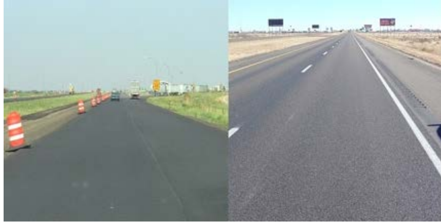
FIGURE 37 Road Condition after Construction.
