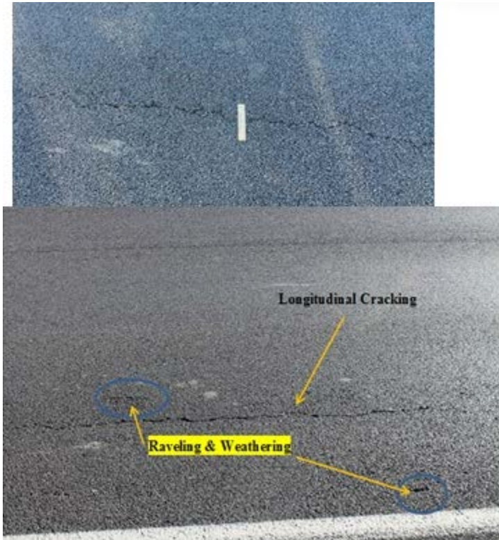
FIGURE 18 Longitudinal Cracking.
