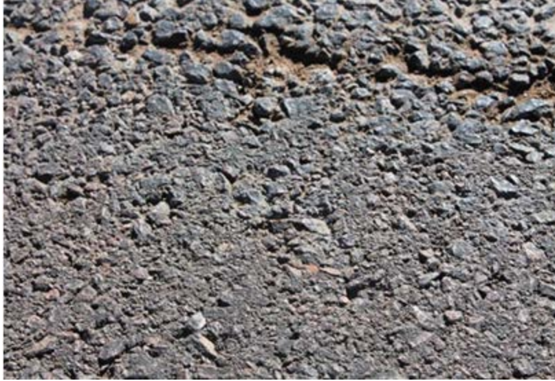
FIGURE 25 Moisture Stripping.
