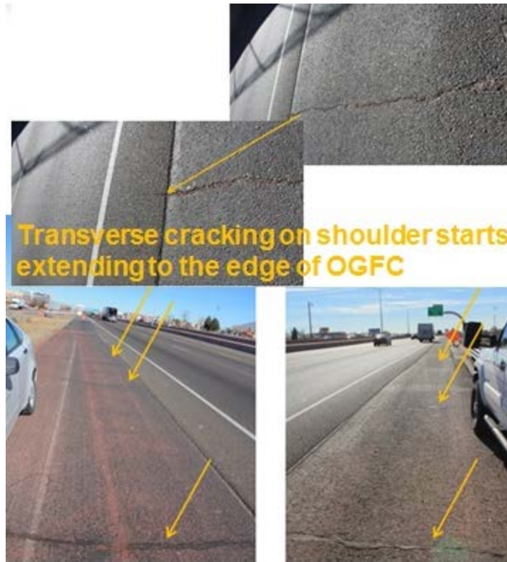
FIGURE 13 Transverse Cracking on Shoulders.
