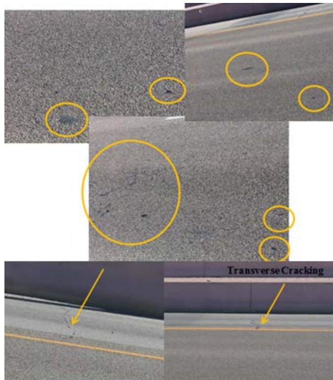
FIGURE 12 Binder Balls.
