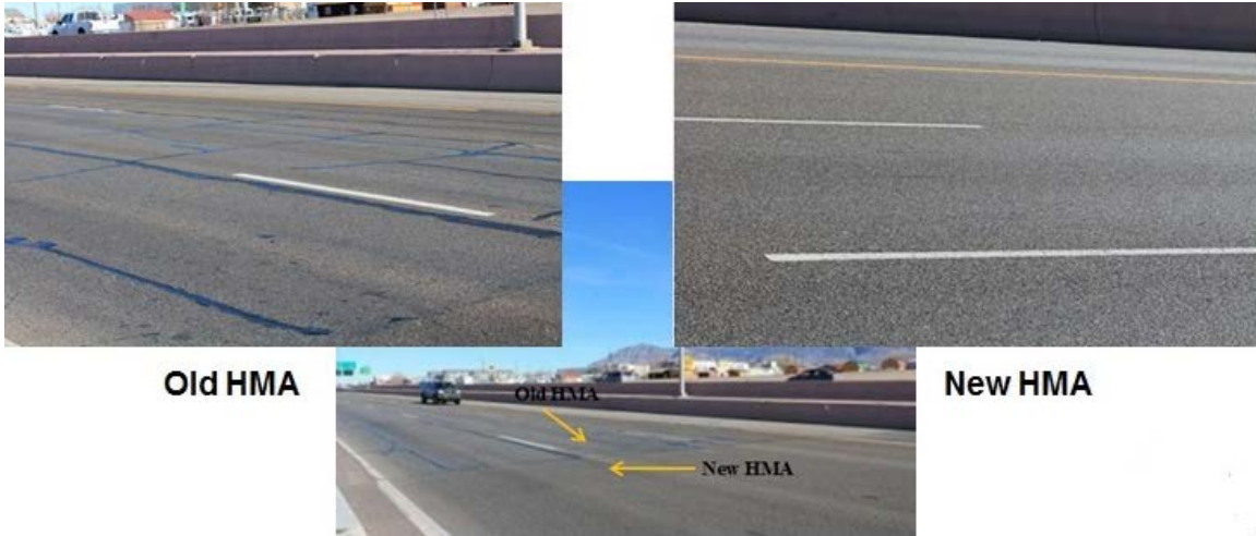
FIGURE 11 General Pavement Condition of the HMA Control Project.
