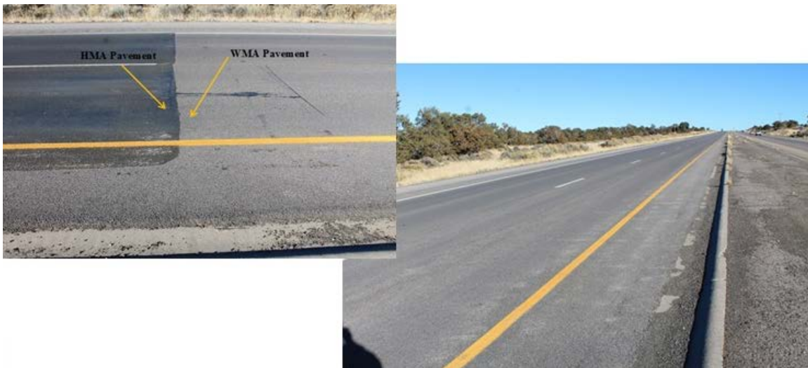
FIGURE 15 General Pavement Condition of the WMA Project.
