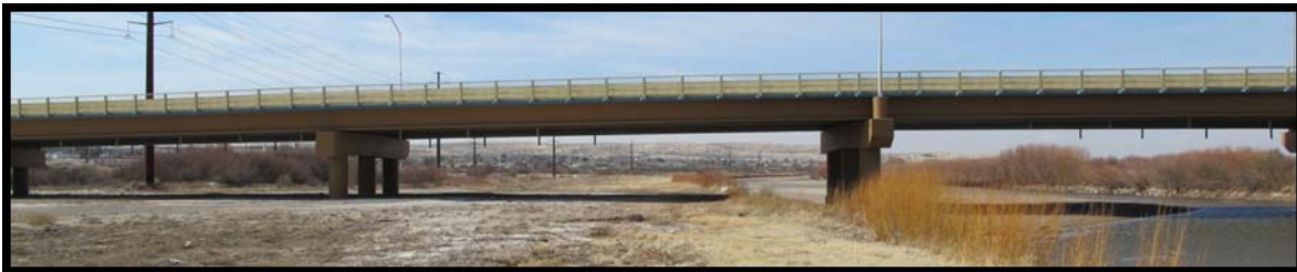
FIGURE 4.6 Three-Span Unit of Sunland Park River Crossing.
