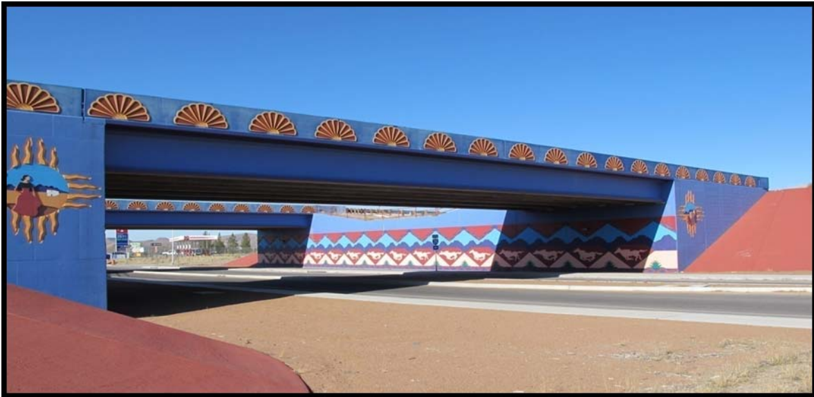
FIGURE 4.1 North Bound Structure of I-25/Doña Ana Interchange.
