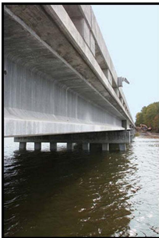
FIGURE 3.12 Second Bridge Built with UHPC in Richmond County, Virginia.
