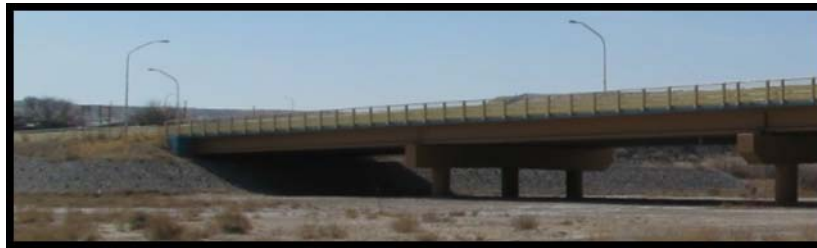
FIGURE 4.5 Two Span Unit of Sunland Park River Crossing.
