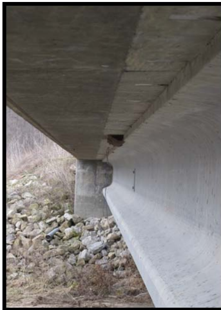
FIGURE 3.4 Girder and Deck Overhang, Mars Hill Bridge.
