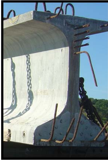
FIGURE 3.7 Strands and Lifting Devices for BTCIO.
