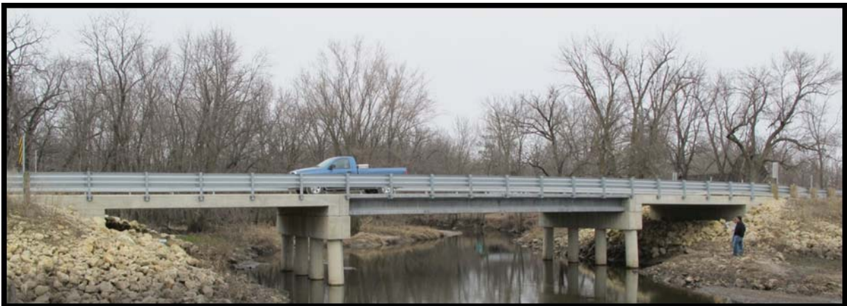
FIGURE 2.3 PI-Girder Bridge in Buchanan County Iowa.
