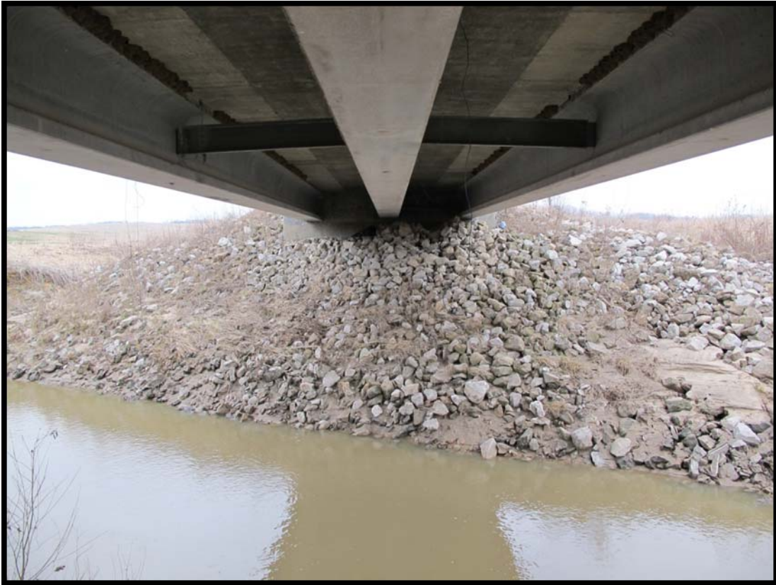
FIGURE 3.3 Underside of Mars Hill Bridge.
